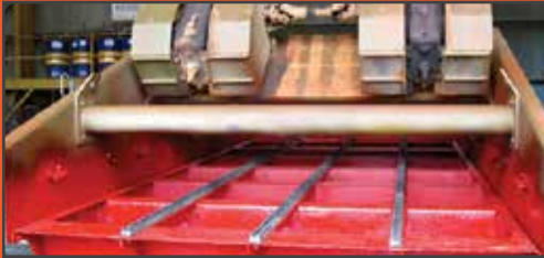
PC Spray - Corrosion and wear protection to a vibratory screen
